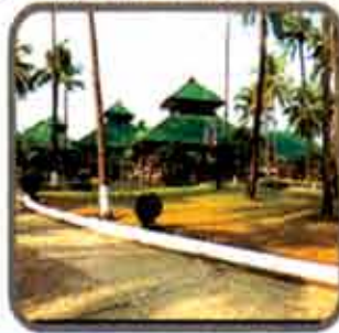
Central Hotel (Ngwe Saung) Project
